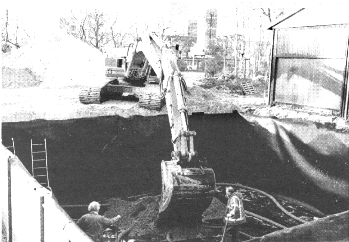
Figure 3.9 Installation of the drainage system in the wooden box.
